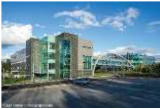
UAA Engineering Building
